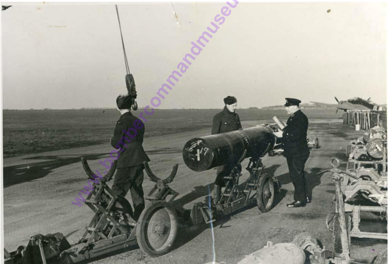
Sea mining, known popularly as 'gardening', was a routine operation for 83 Sqn throughout the war, as Allied forces sought to deny the Kriegsmarine the freedom to roam the seas around Western Europe. This sequence shows a mine being lifted onto a trolley, fused by a Royal Navy armorer and then prepared for loading onto an aircraft. A Hampden waits patiently in the background for its consignment of these effective but unsung weapons.
