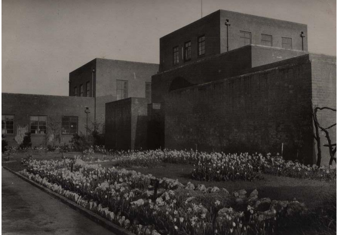
Above left: RAF Scampton Operations Block showing the Hollow Blast Wall surrounding Ops Rooms. Right: Flying Control at Scampton during 83 Squadron's residency. Below: They also served... WAAF's from Flying Control at Scampton.
