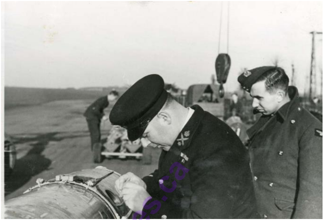
Sea mining, known popularly as 'gardening', was a routine operation for 83 Sqn throughout the war, as Allied forces sought to deny the Kriegsmarine the freedom to roam the seas around Western Europe. This sequence shows a mine being lifted onto a trolley, fused by a Royal Navy armorer and then prepared for loading onto an aircraft. A Hampden waits patiently in the background for its consignment of these effective but unsung weapons.
