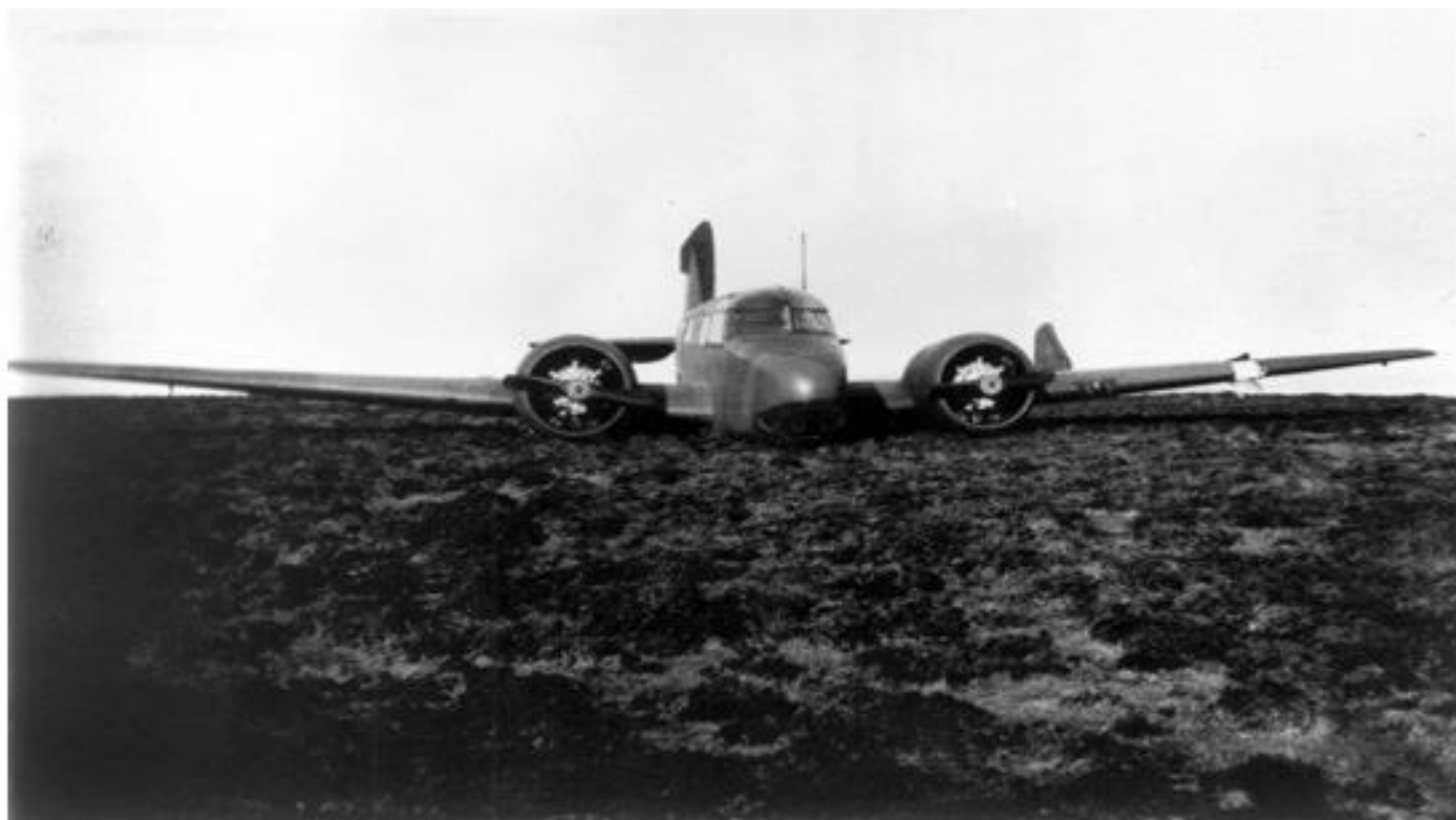
Airspeed 'Oxford' –V3631 – after emergency landing on Auskerry Island Pilot F/S Donald Franko RCAF. Little damage to the aircraft; wooden propellers broken. (photo by Lighthouse Keeper, George Mainland - Dec. 17, 1943)
