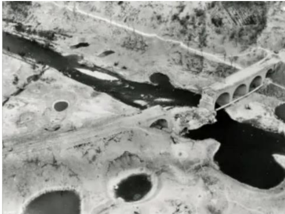
Damaged Arnsberg bridge
