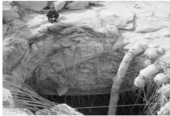
Damage by one Grand Slam on U-boat Pen
