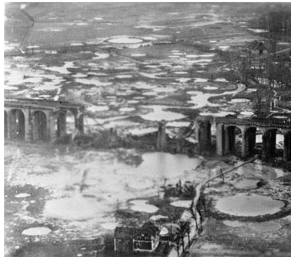
Bomb Damage at Bielefeld Viaduct
