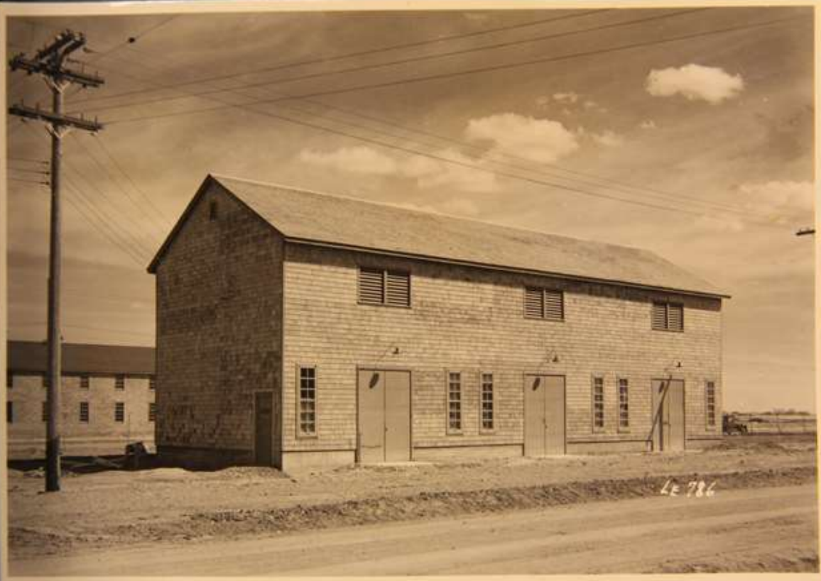
NEW G.I.S. TURRET BUILDING
