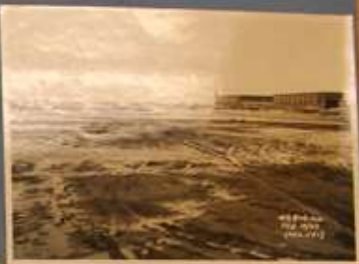
NEW CONSTRUCTION ON BARRACKS 1943
