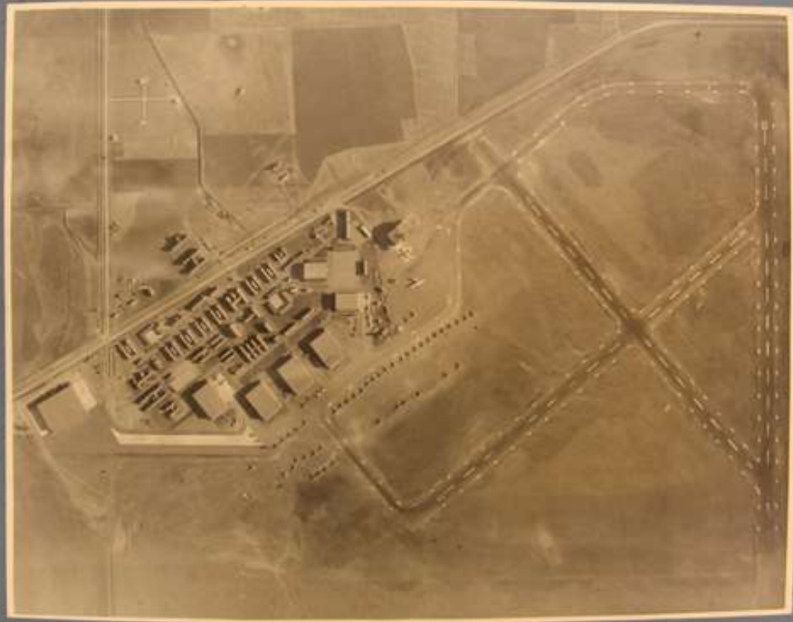
AERIAL VIEW No. 8 - B. & G. SCHOOL ... Dec. 10th, 1947.
