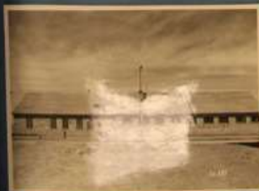
NEW CONSTRUCTION BARRACKS
