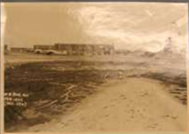
NEW CONSTRUCTION ON BARRACKS 1943
