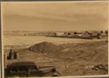
CONSTRUCTION ON NEW BARRACKS
