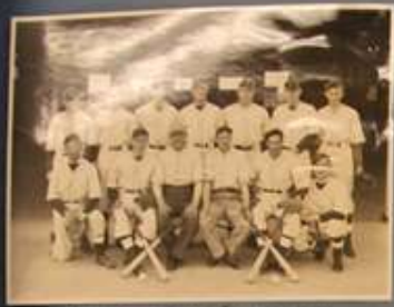
Public Works Administration - July 1942
