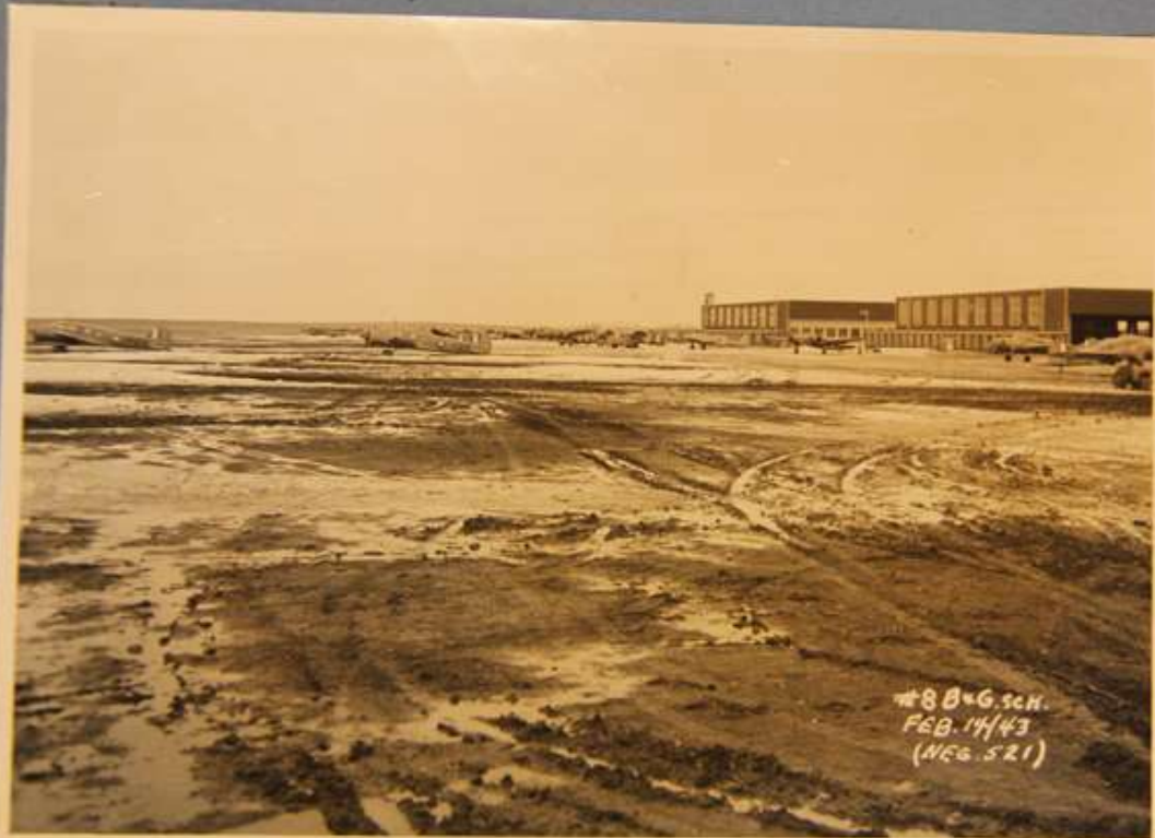
MUD CONDITIONS ON PARKING STRIP
