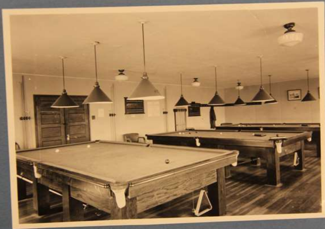
~ DRILL HALL - BILLIARD ROOM ~
