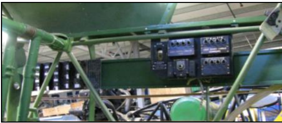
Some of the electrical panels restored
