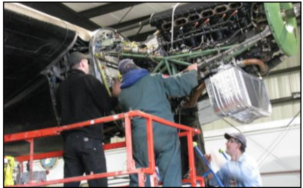
While Ben holds it in place with his hoist, Greg Morrison, and Shane Chipchase secure the attach bolts on one side while Brian Taylor (hidden behind the engine) installs them on the other side with Derek Squire in the lower right assisting.
