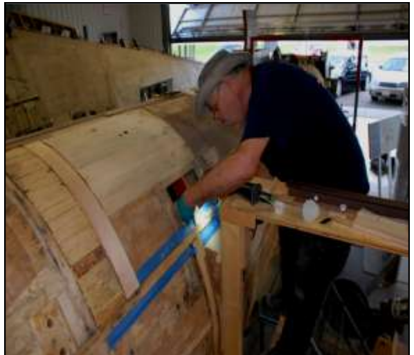
Seen here is one area of the fuselage where "de-skinning" has taken place to deal with water damage, dry rot and shabby repairs from an earlier restoration where the wrong materials were used.
