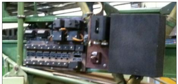
Anson electric panel is mounted in place.
