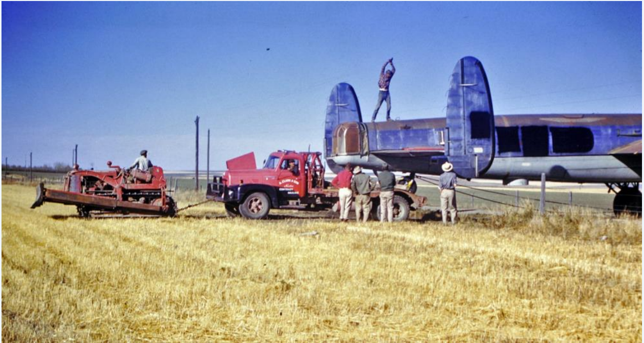
1960 –Under a wire and through a ditch
